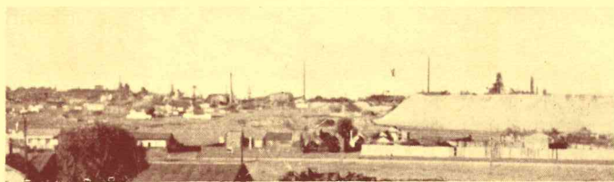
A view of part of "The Golden Mile" taken from the top of the cooling tower of the new power station.
